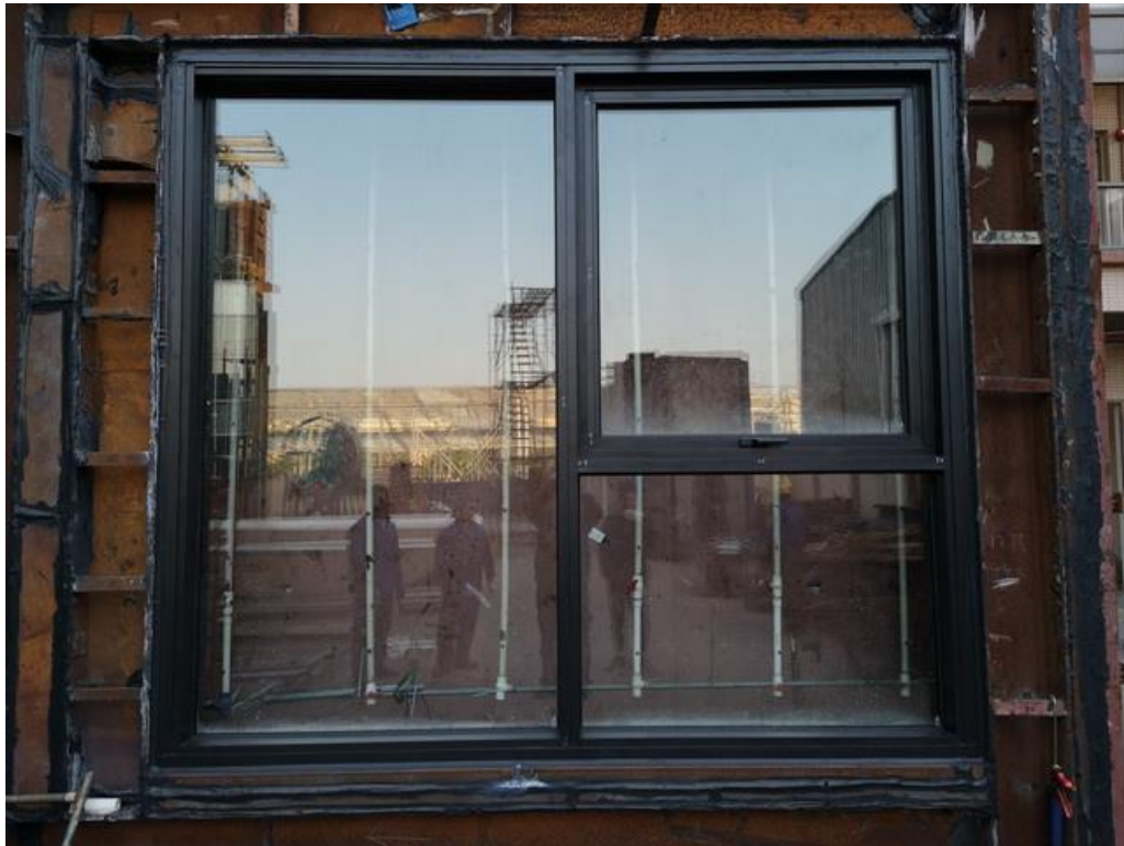
Photo 1: Mock-up of the Window Wall System 150D
