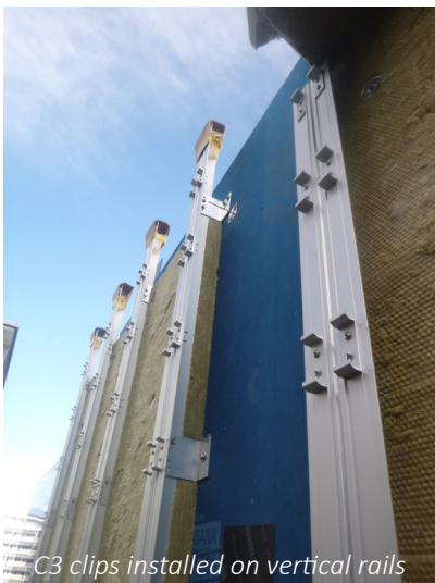
Wind load support bracket
