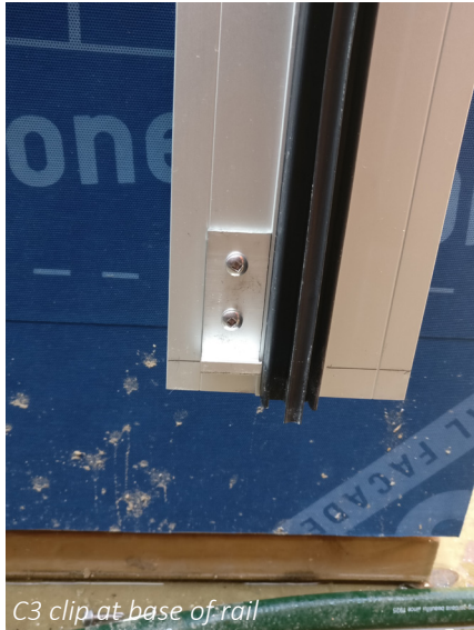
Dead load support bracket
