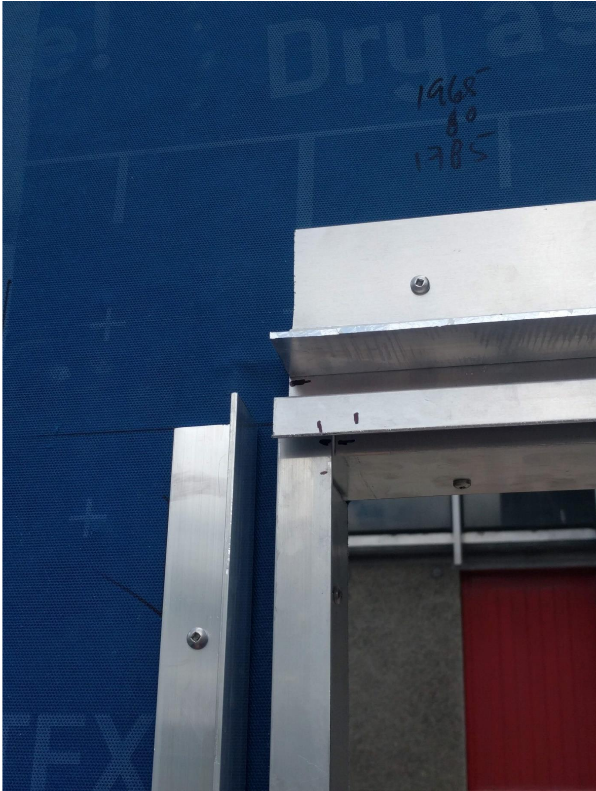
Photo 10: Combustion chamber opening Panel fixing rails, Head flashing and Joinery angles
