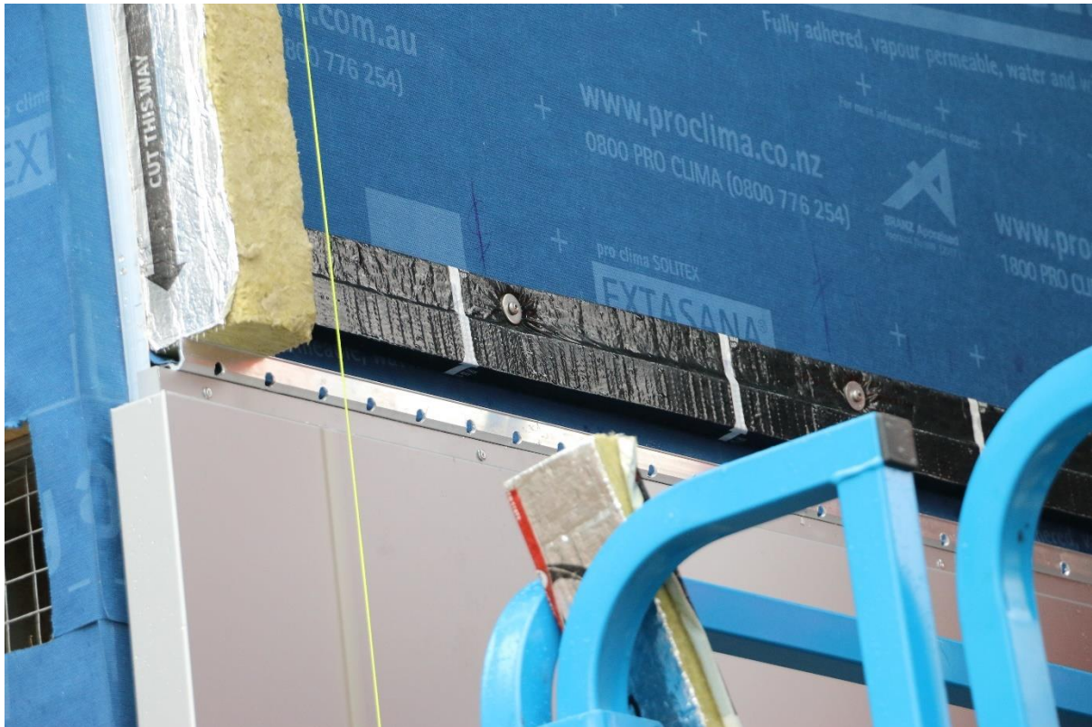
Photo 13: Fire cavity barriers at drainage cavity
