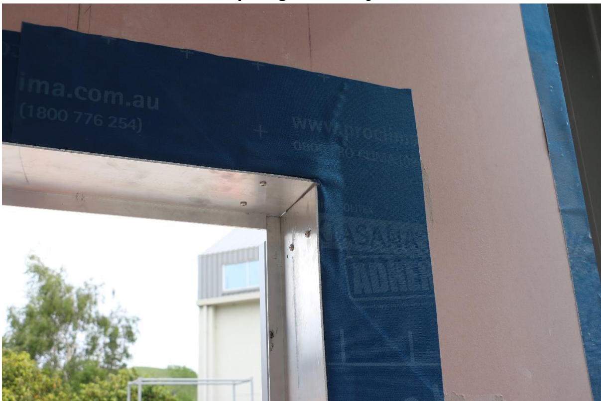
Photo 4: Combustion chamber opening – internal junction
