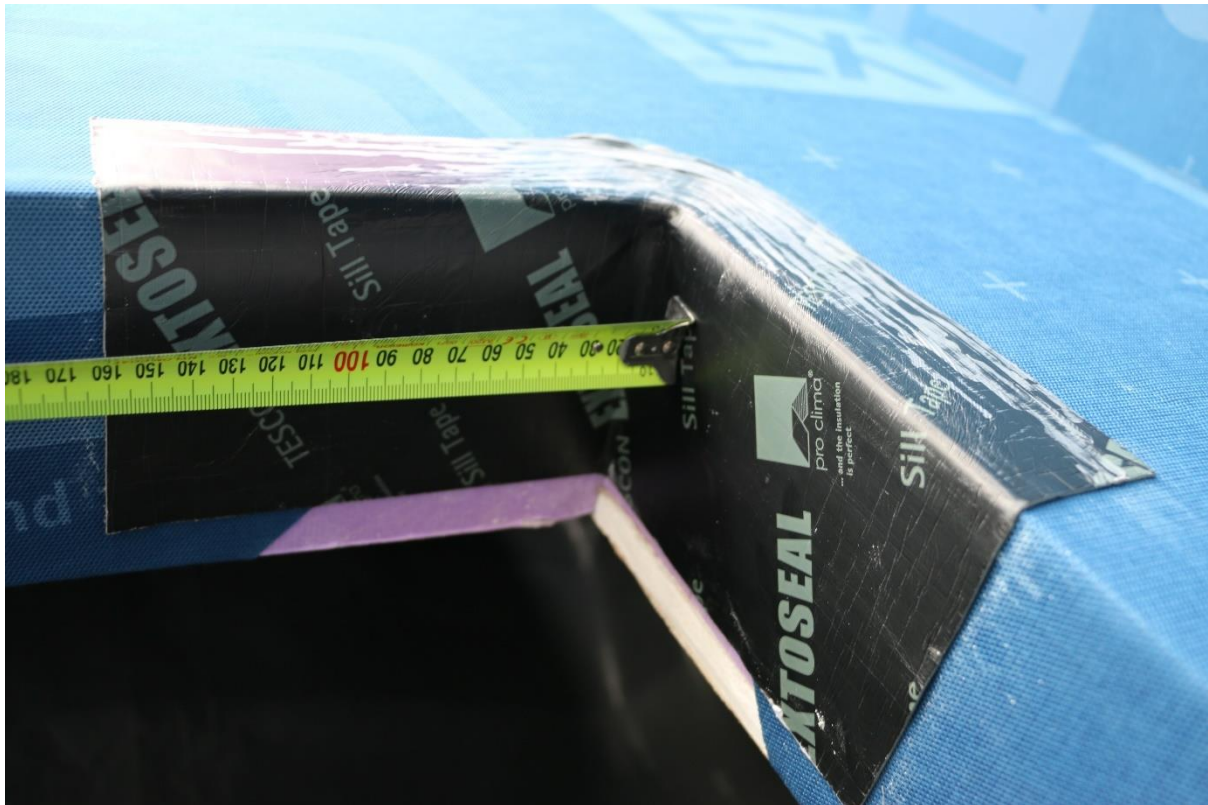
Photo 6: Combustion chamber opening sill tape
