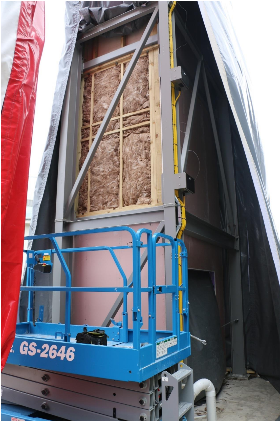
Photo 15: Insulation and Internal lining
