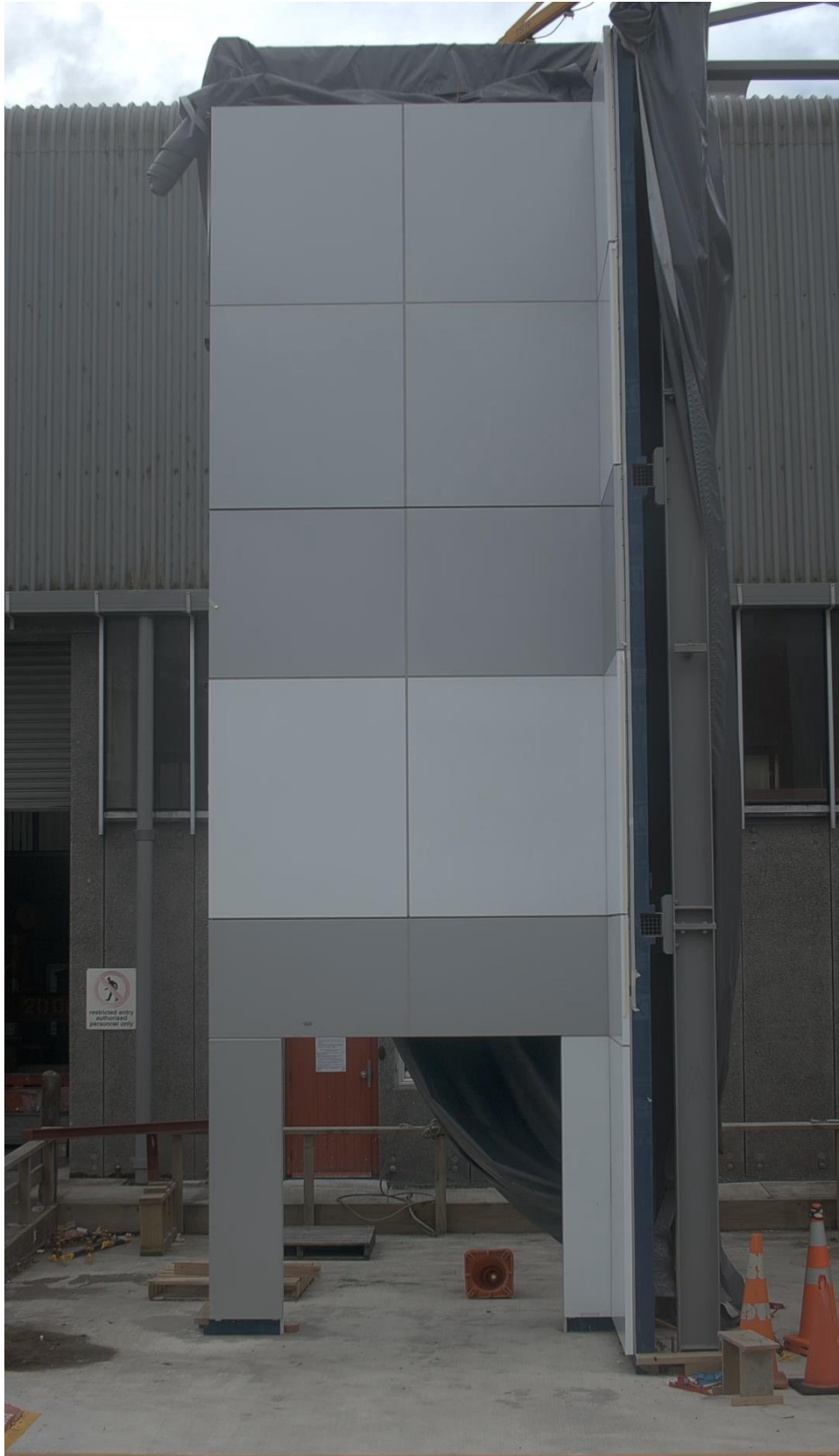
Photo 9: Alucolux panels with sealant applied to junctions
