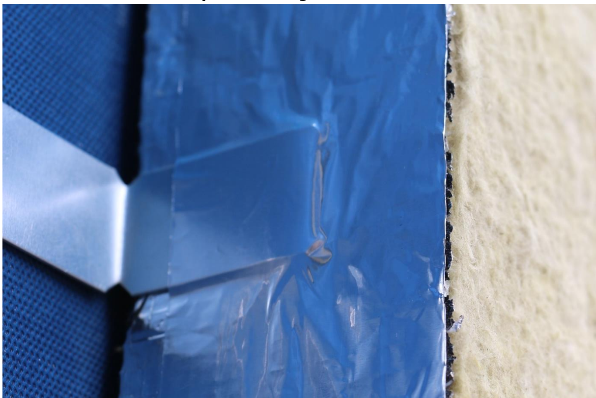
Photo 14: Vertical fire cavity barrier fixing bracket
