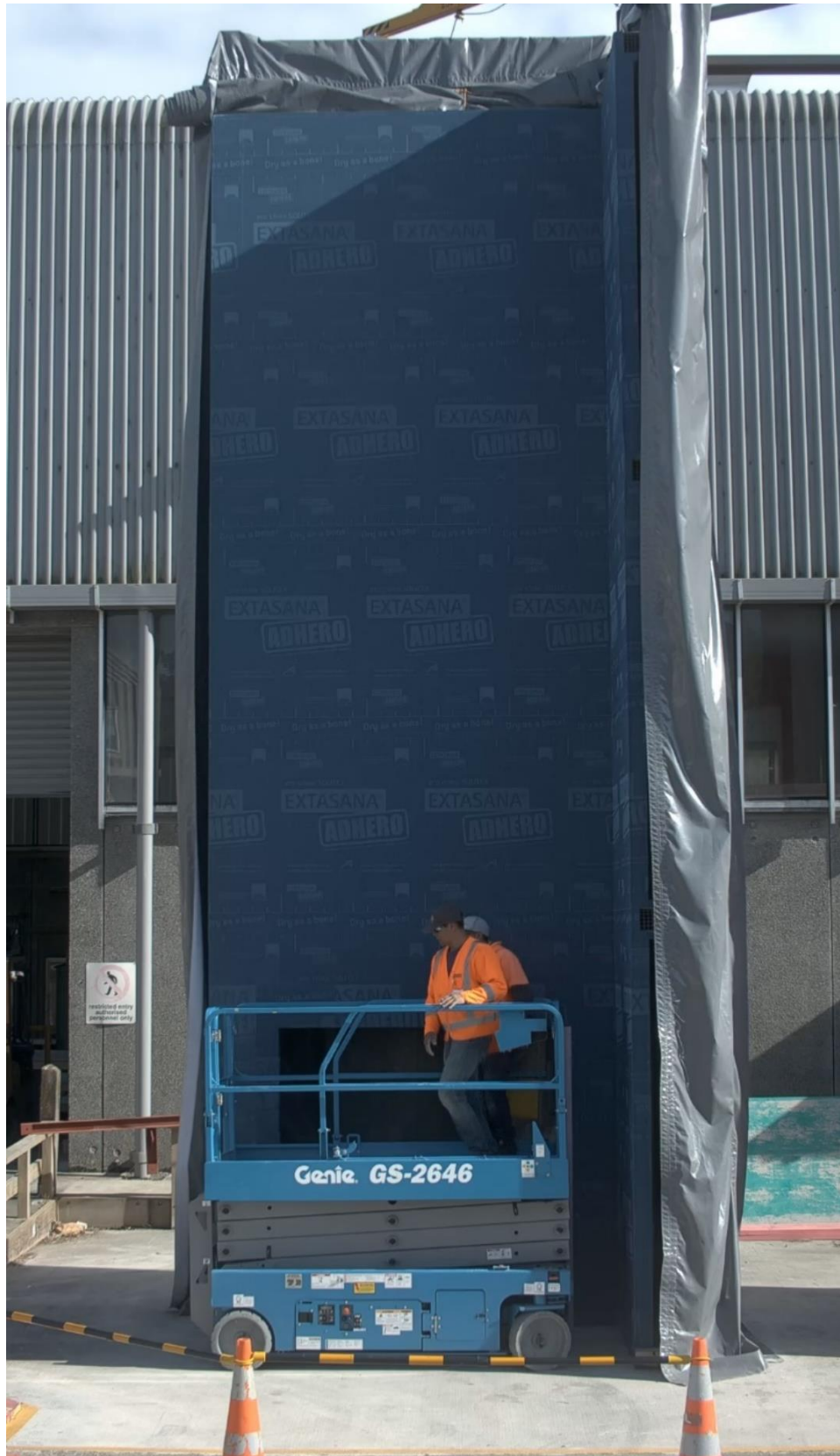
Photo 5: Waterproofing membrane
