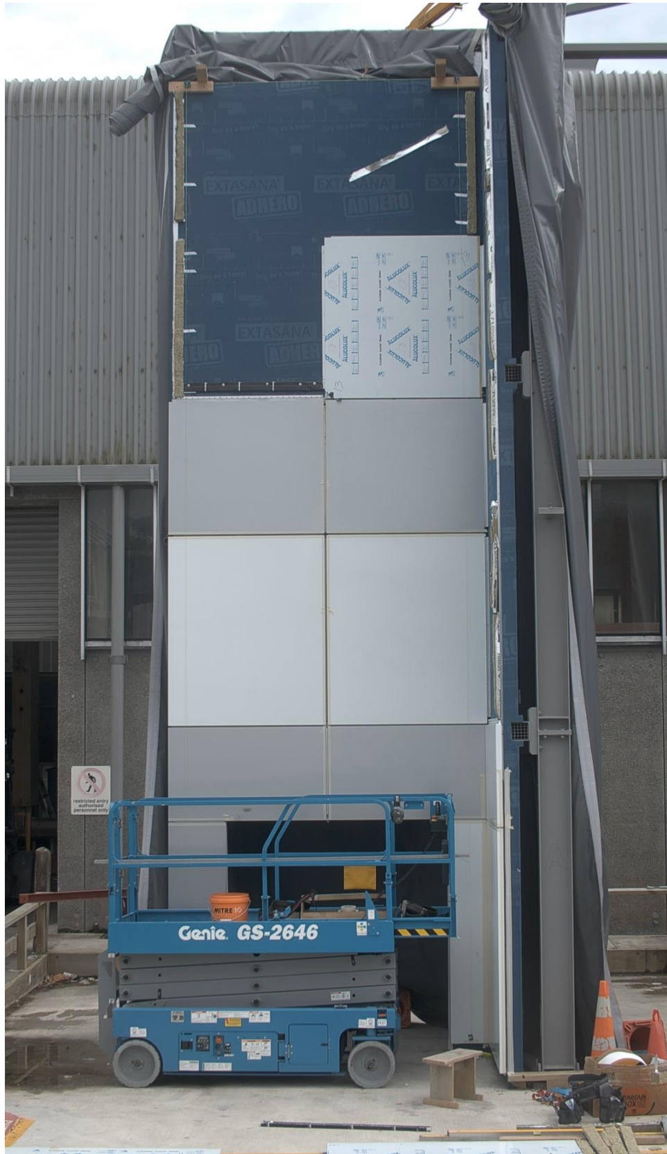
Photo 8: Alucolux panels and fire cavity barriers
