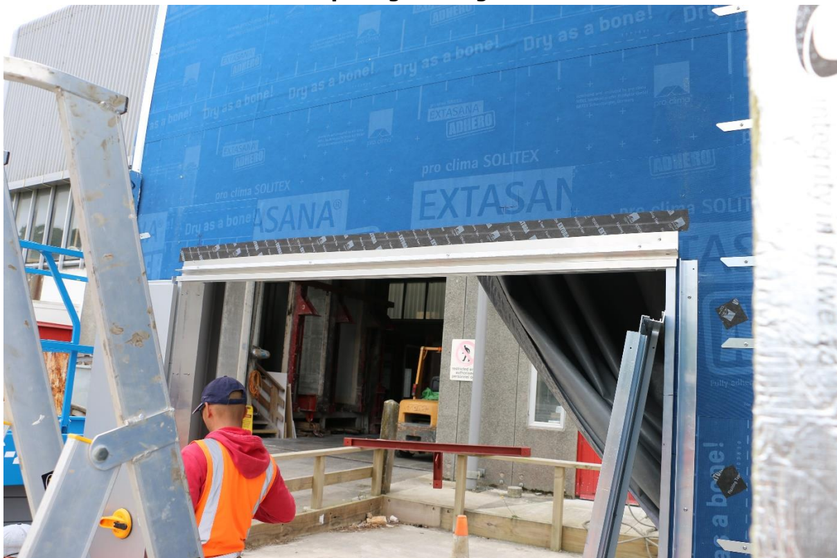
Photo 7: Combustion chamber opening flashing
