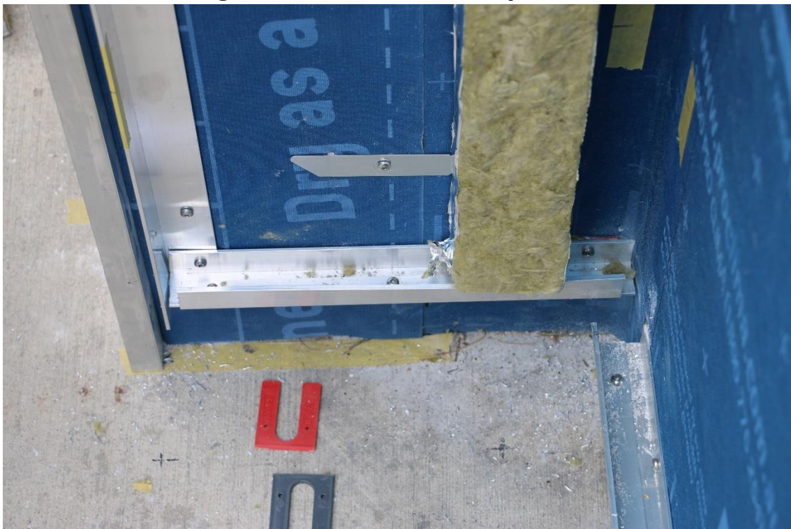
Photo 12: Panel fixing rails and Vertical fire cavity barrier
