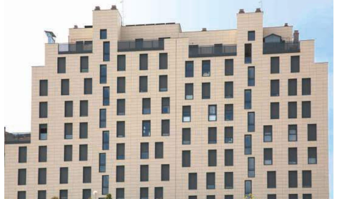
Madrid (SPAIN) Housing block
