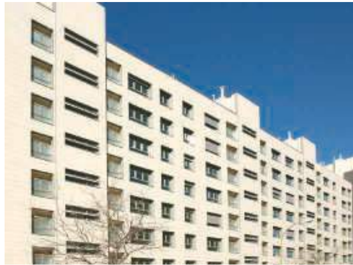
Madrid (SPAIN) Housing block
